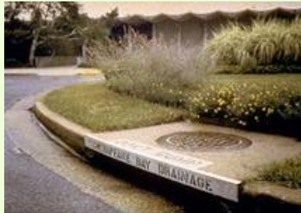
Storm drains can be labeled with stencils to discourage dumping
